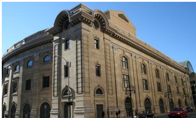
Ellie Caulkins Opera House
